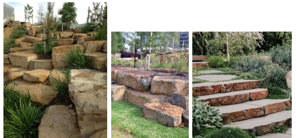
Terracing boulders for retaining and to act as an informal grandstand to MPS Oval Sawn Basalt steps to match natural aesthetic of garden
